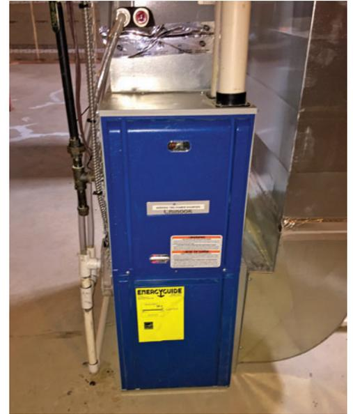
In this St. Thomas, Ont. hybrid application, a small gas furnace and heat pump function seamlessly together
